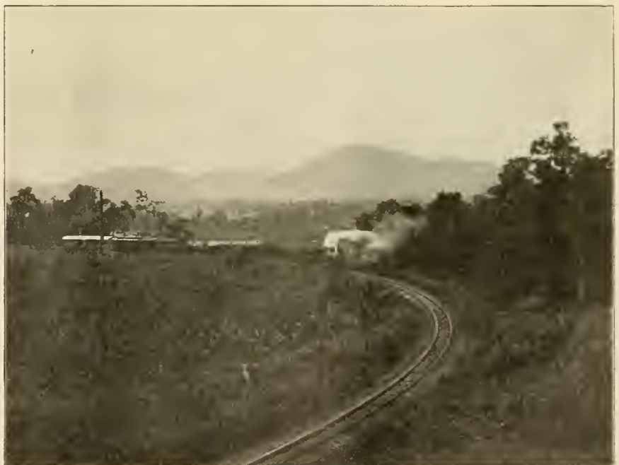
ON THE CAIRNS-KURANDA RAILWAY IN QUEENSLAND, AUSTRALIA.
